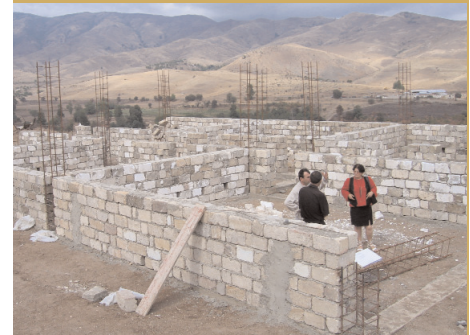
Norashen school construction.
