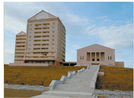
Apartment building and community hall built for war veterans and widows of soldiers who fought in the Karabakh War.
